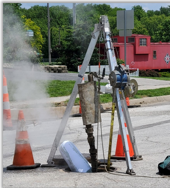
The Cured-In-Place Pipe will help prevent future leaks and root infestation within City sewer lines
