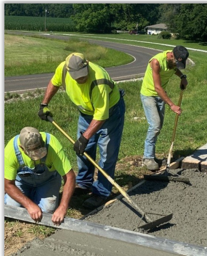
Street maintenance crews repair sidewalk panels in the City
