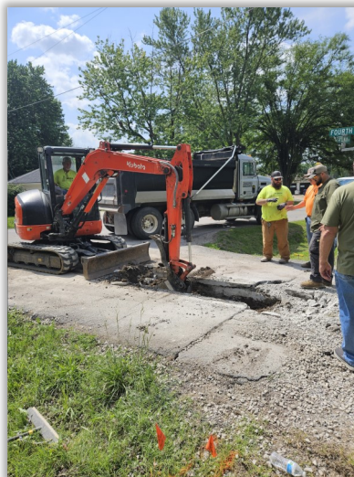
Utility contractors make waterline repairs (paid from the CWWS Fund)
