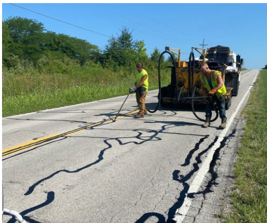
The City partnered with Asphaltic Surfaces for the completion of the 2025 Street Maintenance Program which includes milling and overlaying Commercial Avenue to extend the roadway's service life.
